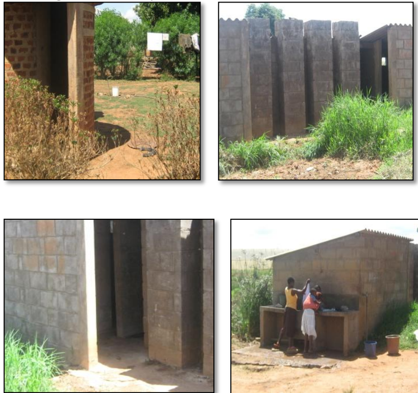
Figure 10: Sanitary Facilities at Kara Farm
