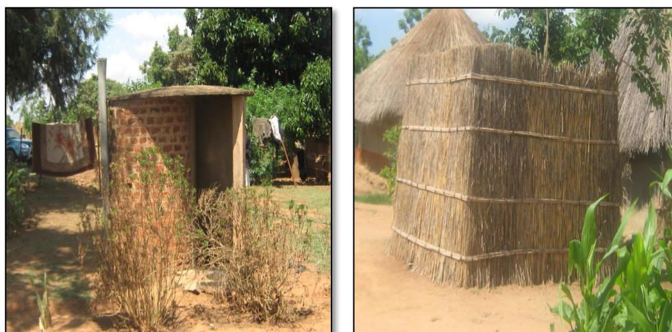
Figure 12: The Old and the New Toilets for Former Farm Workers at Kara Farm
