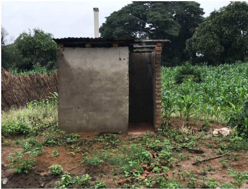
Figure 9: A properly built toilet by one household
