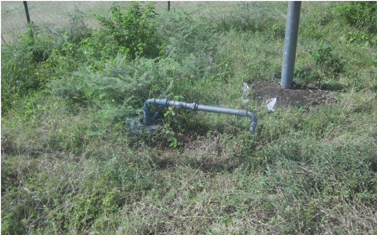
Figure 5: Photograph of a borehole constructed by the Ministry of Water that has clean water but does not function
