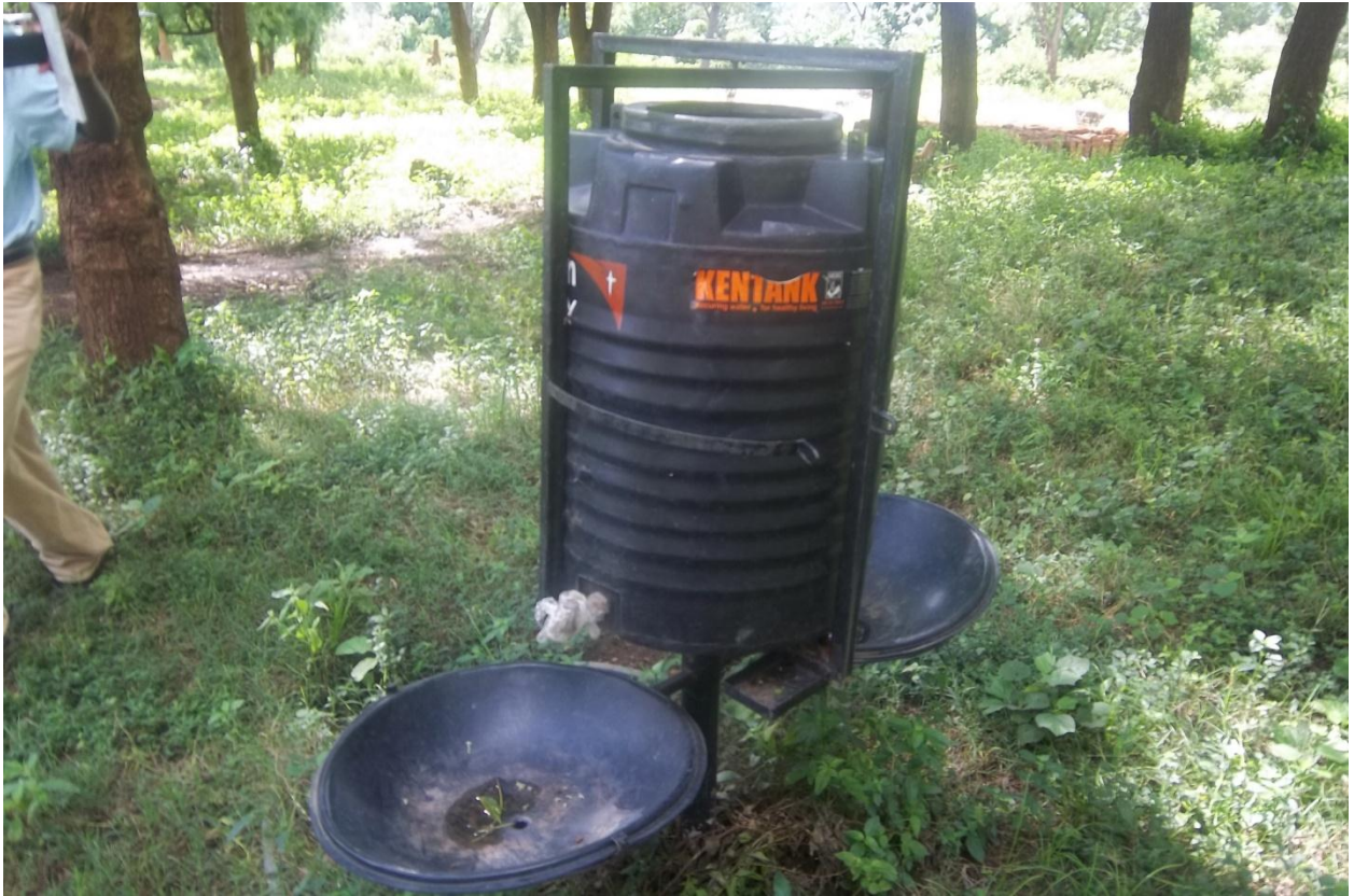
Figure 4: Photograph of hand-washing equipment donated by World Vision International to Chepkum Primary School which is not functioning due to the lack of water
