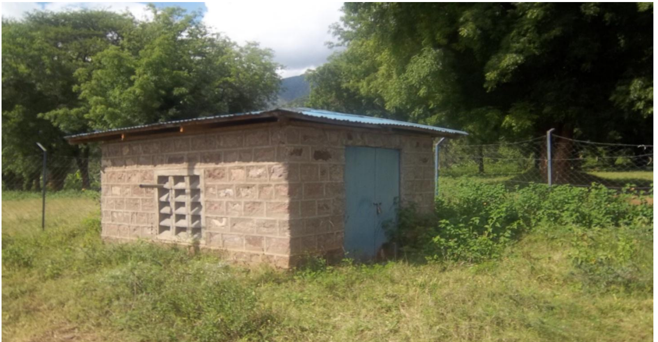
Figure 7: Photograph of a borehole which was constructed and drilled by the World Vision International (WVI). It has clean water but is not functioning.
