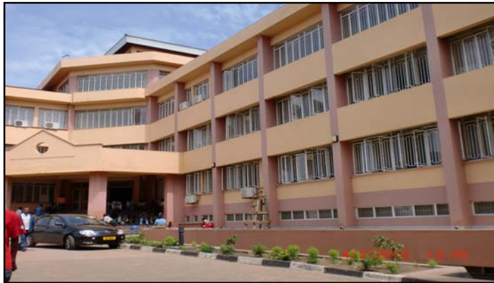
Picture 4: A section of the Limbe Police Station housing the VSU.
