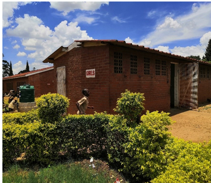
Figure 13: Girls ablutions block with outside water tank
