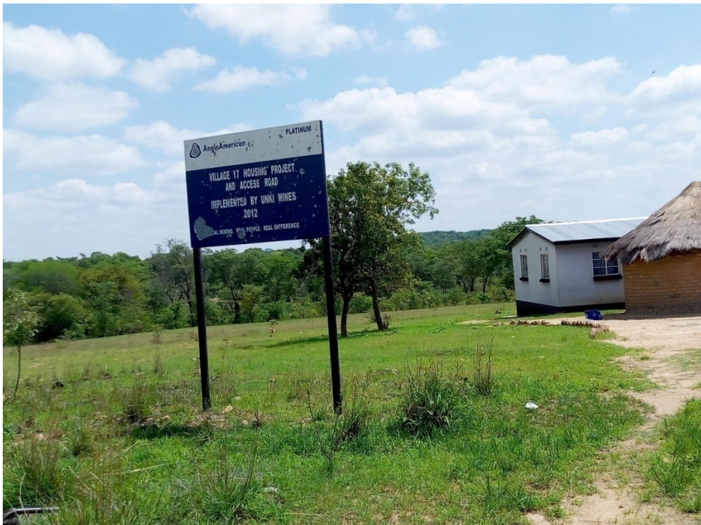
Figure 4: Photograph of a three-bedroomed house built in Village 17 by Unki Mine in 2012
