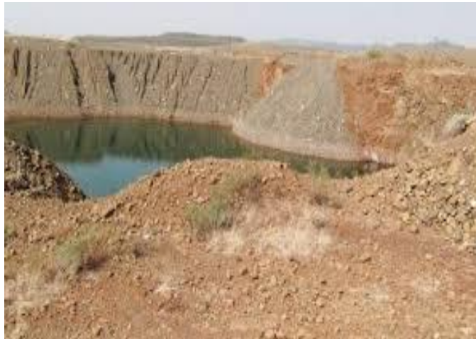
Figure 1: Photograph of a huge open mine pit in the raining season which has not been filled after the cessation of mining operations.
