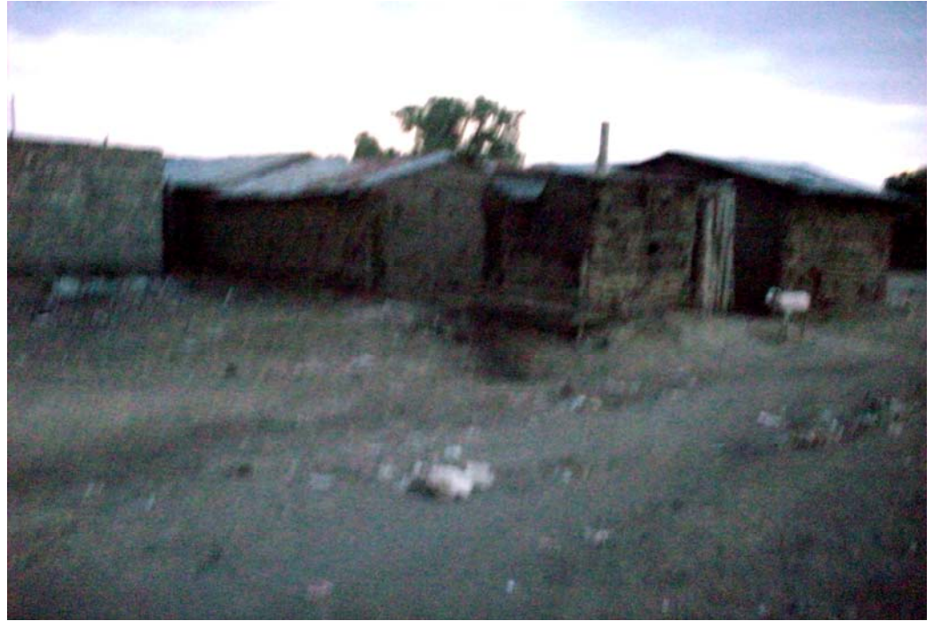
These are semi-permanent structures with mud walls and an earth floor in Karagita
