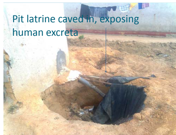
Figure 13: Photograph of a shallow collapsed pit latrine
