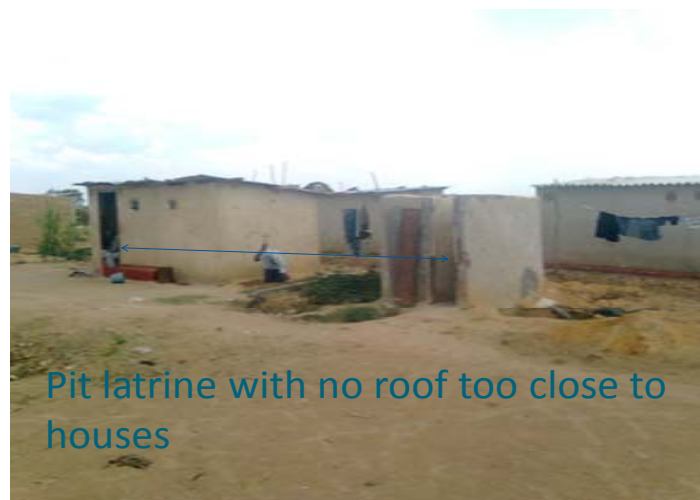
Figure 14: Photograph of pit latrines which do not have roofs and which are too close to nearby homes and wells whose water they may contaminate
