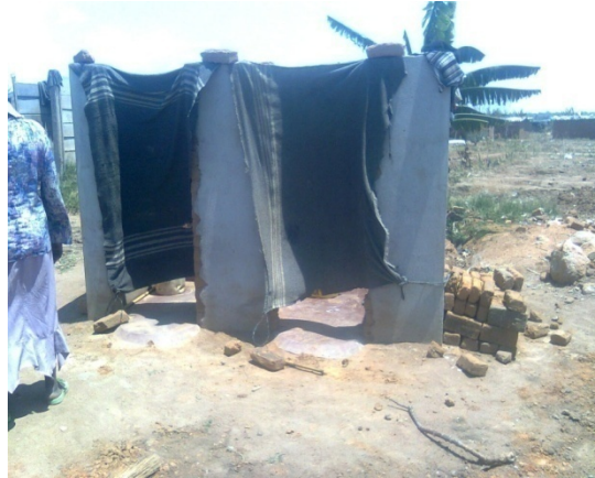
Figure 13: Photograph of a shallow collapsed pit latrine
