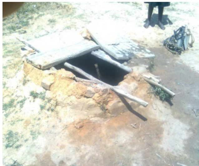
Figure 1: Photograph of an unprotected well
