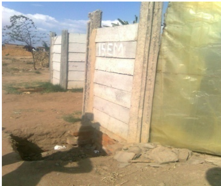
Figure 3: Photograph of an open pit latrine without a door or roof
